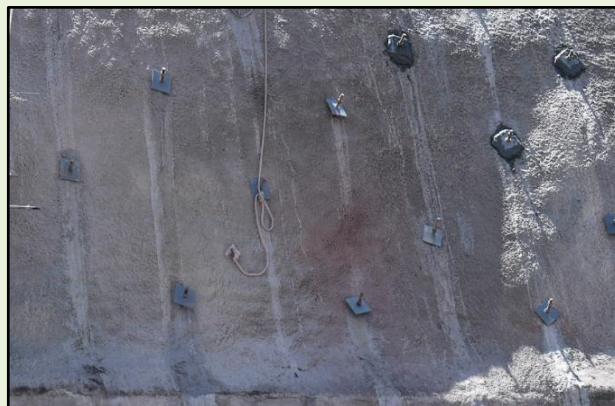
Figure 68: Ground Anchor Wall with Riprap and Shotcrete Slope Stabilization
