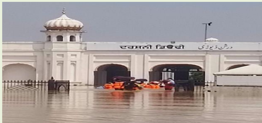
Figure 16: Flooding at Kartarpur Corridor, Narowal Due to Inadequate Drainage Infrastructure
