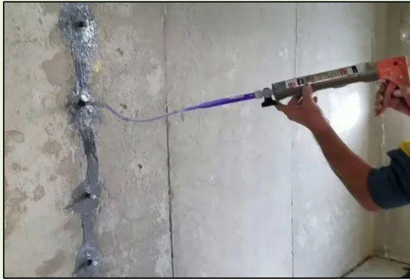
Figure 63: Epoxy Injection for Structural Crack Rehabilitation
