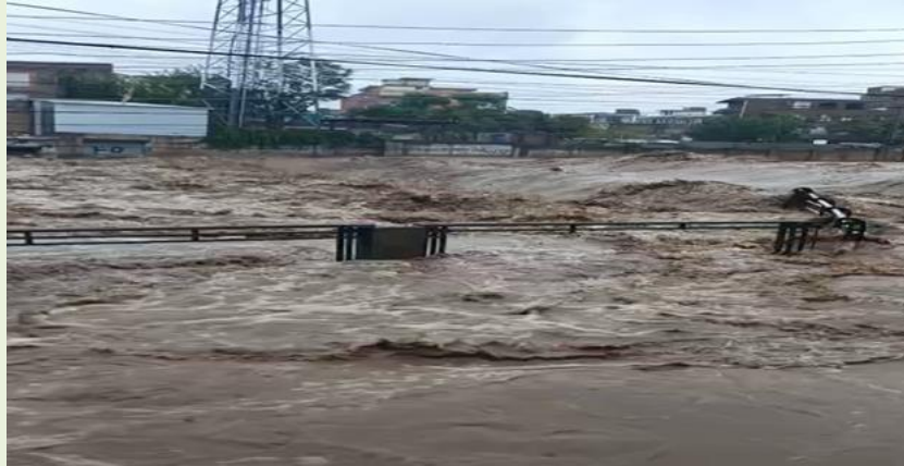
Figure 7: Severe Urban Flooding Due to Inadequate Drainage Infrastructure
