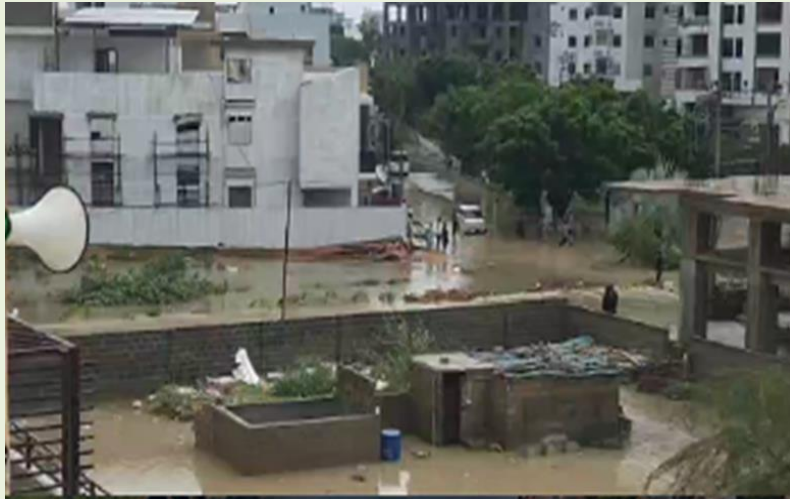
Figure 27: Building Collapse in Karachi due to Heavy and Persistent Rainfall
