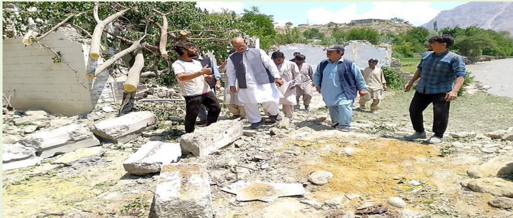
Figure 4: Ground Instability and Vegetation Uprooting in Chitral
