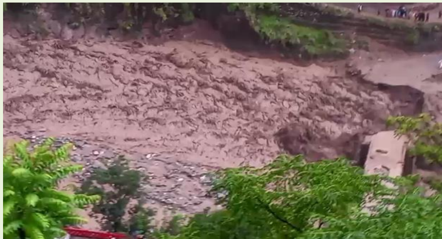
Figure 43: Bridge Collapse in Neelum Due to Flood-Induced Structural Failure
