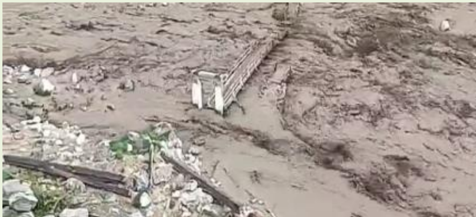
Figure 35: Bridge Collapse at Babusar–Chilas Following Cloud Burst
