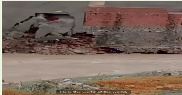
Figure 14: Structural Failure of Residential Building Due to Foundation Settlement and Erosion
