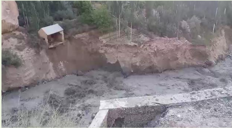
Figure 34: Riverbank Erosion and Slope Failure at Shishper Following GLOF Event
