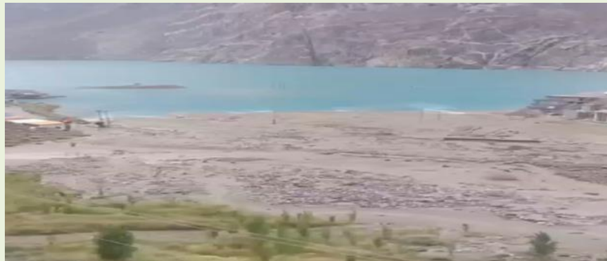
Figure 33: Road Damage at Brundubar Nullah, Hunza – Result of Inadequate Design
